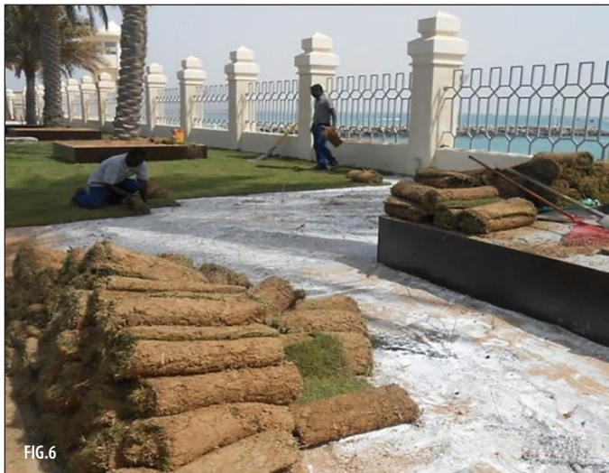
Landscape workers apply a layer of perlite before spreading turf in order to increase water-holding capacity of the soil. (Courtesy of Gulf Perlite)
