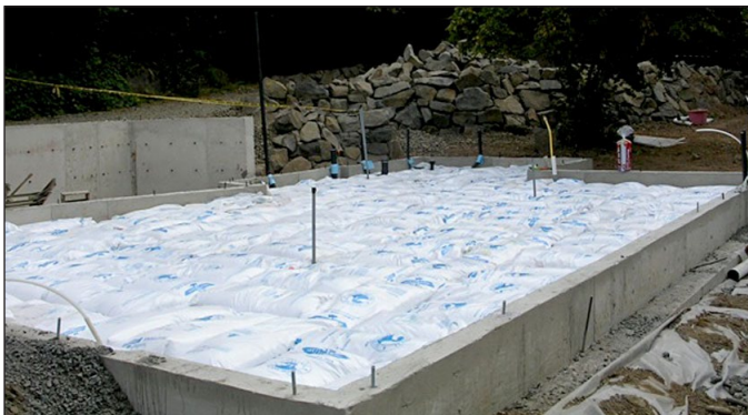
Top: placing unopened perlite bags on grade.
